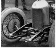
Miller-Durant 183 left, Miller-Durant 122 right, with identical 1882-A front spring horn brackets. Note the rounded radiator shells on both.
